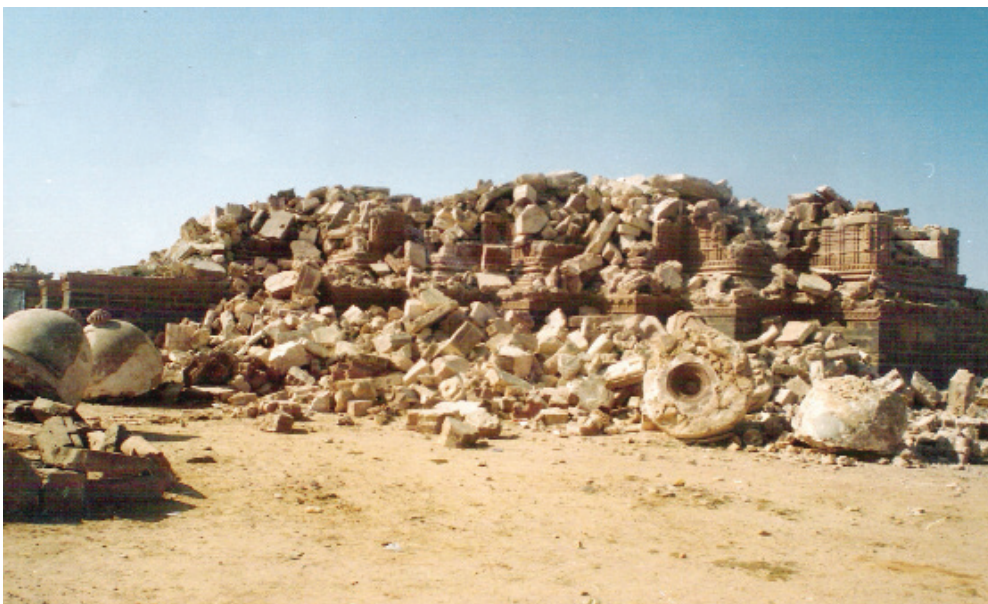
The historical Lakhpatji Chaturdi monument lies in ruins after the earthquake in 2001.
