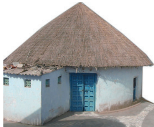
Changing face of the Bhunga - After the earthquake, traditional mud Bhungas have been replaced by brick Bhunga-type structures.
